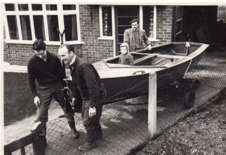
Finished hull on trailer, Nick Mills, Jim Naden, Derek King & Son
